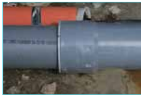
RESULT: FULLY RESTORED DUCT
