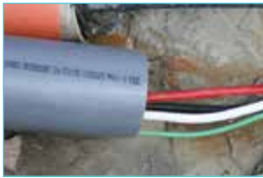
CUT DUCT AS PER EPR KIT INSTRUCTIONS
