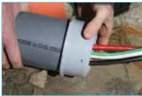
CEMENT ADAPTER ONTO DUCT
