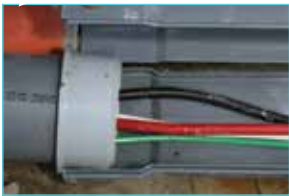
CEMENT EPR KIT INTO PLACE
