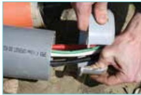
OPEN ADAPTER AROUND CABLES
