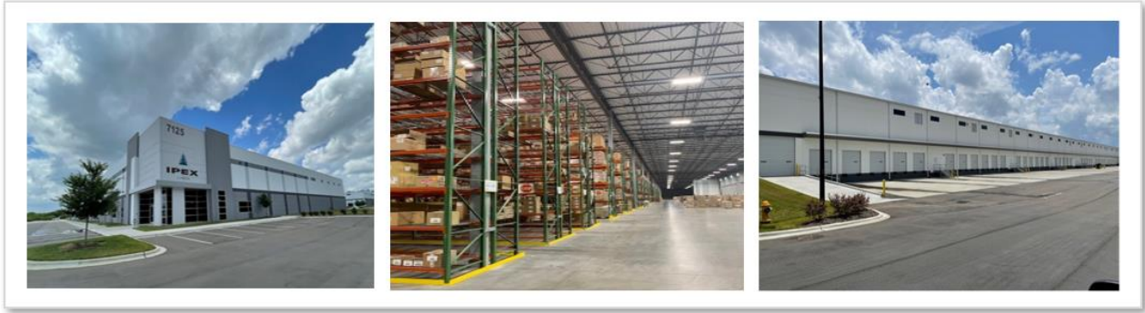
IPEX's distribution centre in Charlotte, North Carolina
