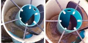
flow energy to suppress the turbulence which releases the noxious gases. By installing one Vortex Flow unit, the municipality was able to save the money it would have spent on adding chemicals to manage the H<sub>2</sub>S emissions.
