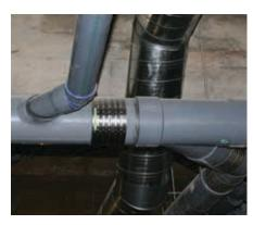
Group/CEC Mechanical, the foreman on the job. "This was our first time using the IPEX (MJ Grey) products, and it was a very easy transition for my team. We would normally have used cast iron pipe for such a large diameter drainage system, but System XFR took fewer people less time and less labour to install."
