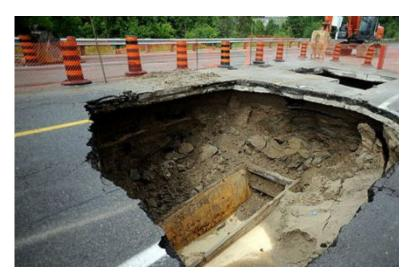
The quality and quantity of flow in a sewage piping system is also a concern for engineers and utility owners. Infiltration into sewer pipes due to leaky joints can drain groundwater levels and/or surrounding surface water, potentially transporting
