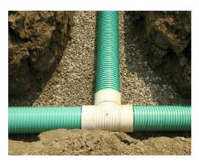
engineers can ensure leak-free joints that are watertight and air-tight by simply specifying sewer pipe and fittings from a single manufacturer with joints that are third-party certified to a hydrostatic pressure of 50 psi and by specifying low-pressure air testing in the field to an air pressure of 5 psi per CSA B182.11.
