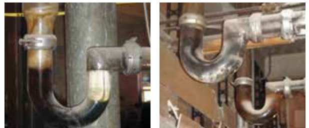
Crud buildup from years of operation are clearly visible in glass waste lines
