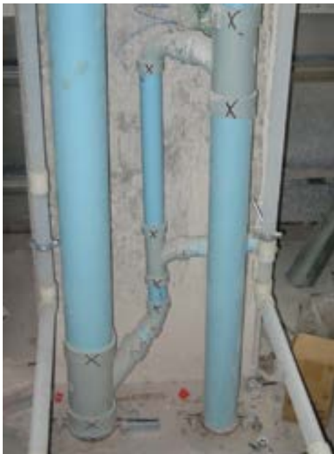
IPEX Labline® & Enpure™ systems being installed
