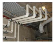
other systems running through the tunnels. Using a double containment system ensures a spill-free system for better reliability."
