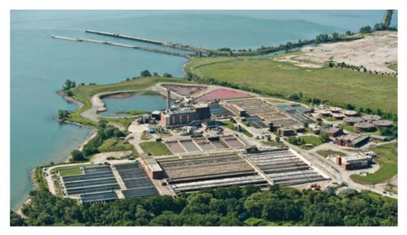
riginally built in the late 1950s to handle an average flow of 2 million gallons per day (mgd), the G.E. Booth (Lakeview) Wastewater Treatment Plant (WWTP) is a key facility for the Region of Peel. In 2009, the facility underwent a \$260 million expansion to treat 137 mgd from the more than 1.3 million residents and 90,000 commercial businesses in the eastern section of Mississauga, Brampton, Bolton, and Caledon East.
