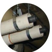
"We chose the PVC Guardian double containment system because it offered the corrosion resistance we needed, and it is was the most cost-effective option," says Petran. "IPEX also worked with us to find the most economical way to design the system with expansion joints to accommodate the seasonal temperature changes in the tunnels. We also liked the fact that IPEX provided a local technical sales representative to work closely with us and the contractor."
