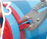
Secure the Pipe Stop using a pair of vice grips.
