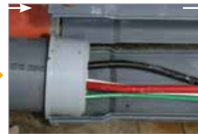
CEMENT EPR KIT INTO PLACE
