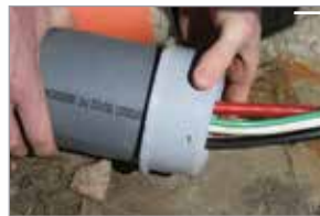
CEMENT ADAPTER ONTO DUCT
