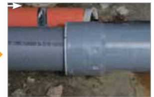
RESULT: FULLY RESTORED DUCT
