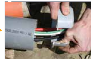
OPEN ADAPTER AROUND CABLES
