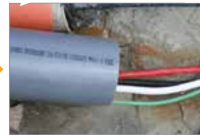
CUT DUCT AS PER EPR KIT INSTRUCTIONS
